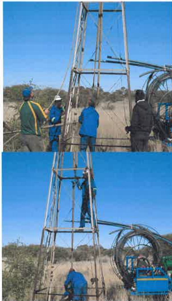
Testing of boreholes at Rust & Vrede Farm, Ms Khantwans Farm
